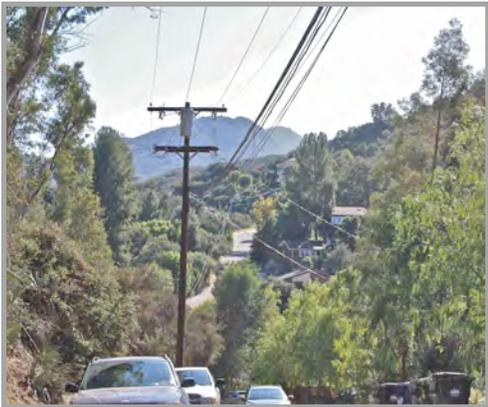
Southern California Edison provides power to the Planning Area through a number of transformers and transmission lines. There are no substations here. Transformers are at risk from fire, potentially knocking out power to areas when they burn or shut down as a result of overheating.<sup>14</sup>
